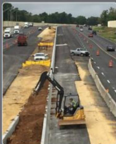
More than **28,000** linear feet of drainage pipe installed.
