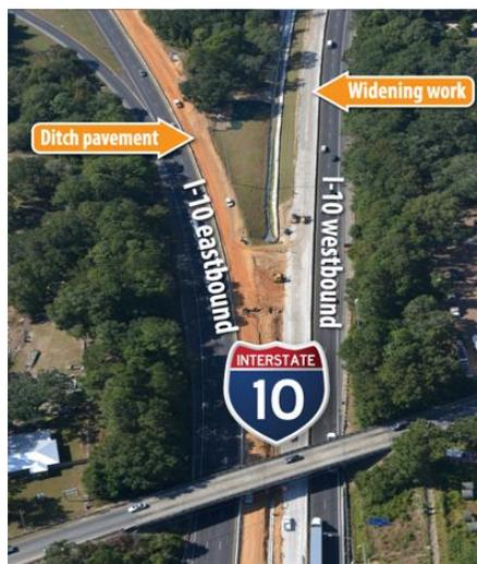
In this area of I-10 east of the U.S. 29 interchange, the construction team is installing the concrete ditch and
