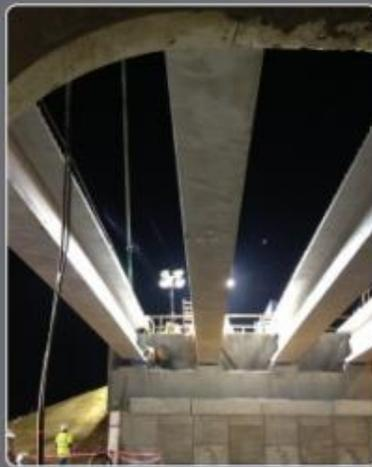
**16** beams installed for the new Scenic Highway overpass. Each weighing approximately **60** tons.
