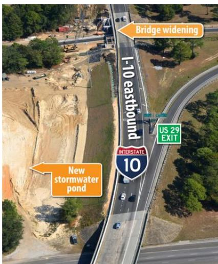
Crews are excavating the area to the left for the new stormwater pond. At the top of the picture,
