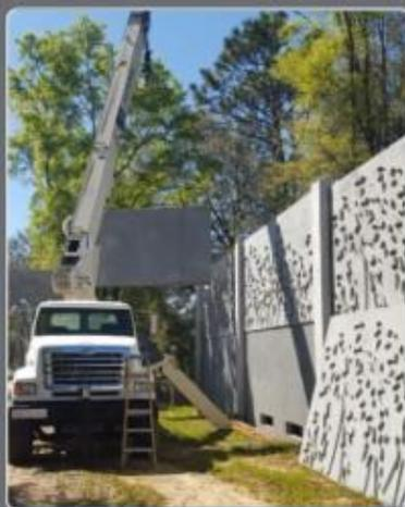
**5** miles of sound walls installed, including **1,800** concrete posts.
