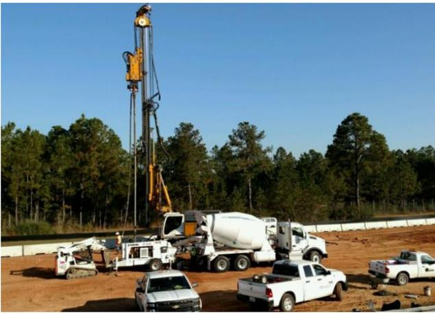
*Crews perform "rigid inclusion work" at the I-10/Avalon Boulevard ramps. This process stabilizes the soil so that it can be built at a higher elevation.*
